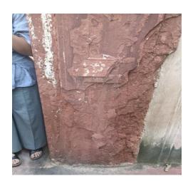
The area of Qudasiya Bagh still has high water table. The layers of sandstone are seen flaking due to Salt accretion or percolation of water and reverse osmosis.
