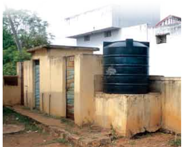
Toilets in a Private Preschool in Andhra Pradesh
